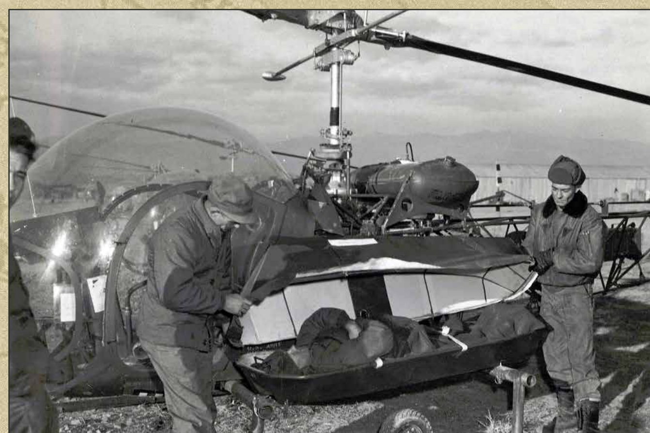
An external litter pod on an H-13 Sioux helicopter. The helicopter was able to carry two litter pods, and these were often fitted with acrylic glass to insulate the medical evacuee from the cold environment. (Courtesy of U.S. Army Medical Department)
